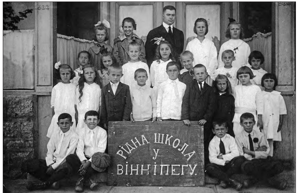
Teacher Yuriy Genyk poses with a class in front of the Ukrainian National Home Association's Ridna Shkola , or heritage school, in this 1916 photo. The building at the corner of Burrows Avenue and McGregor Street is still standing.
